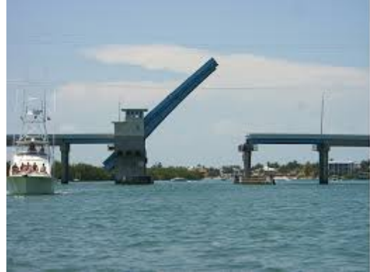
Figure 2 – Drawbridge span raised as one.
