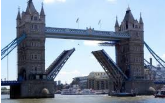
Figure 1 – Drawbridge, span raised as two halves.
